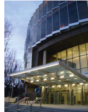
Main entrance structurally glazed canopy
