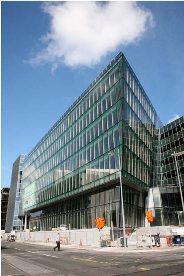
Oblique view on north block overhanging glass corner
