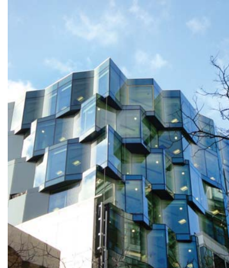
Oblique view - rear elevation
